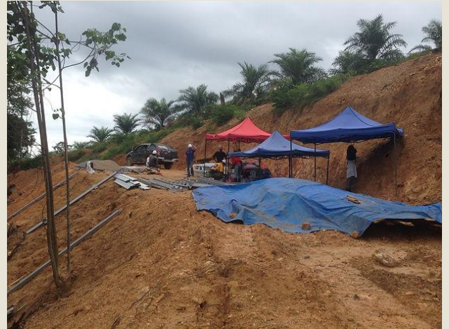
The sloping build site
